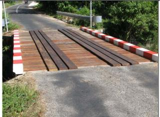
Tanoliu Bridge with the new deck timbers all in place. Work on the Ulei Bridge continues.
