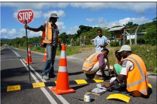
Installing speed bumps in Tanoliu. These are a trial to see how the bumps perform, especially to determine how effective they are at slowing traffic down.
